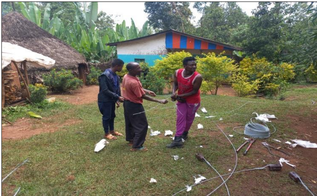
Picture 4 – Conductor Preparation Work in Progress, SNNP Region (No PPE Used)
