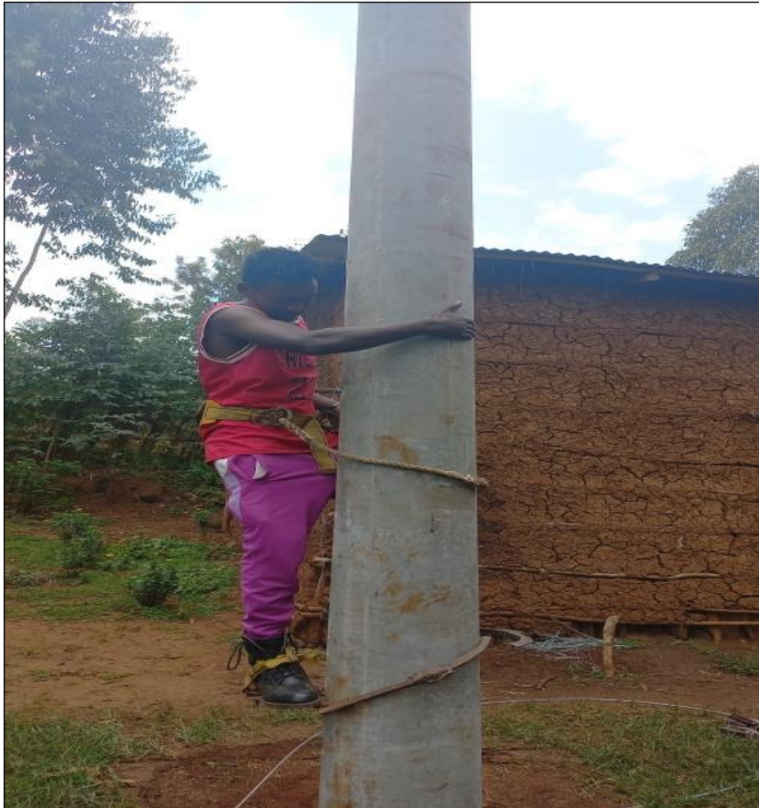
Picture 3 – Worker using Climbing Shoe for Work-at-Height, SNNP Region
