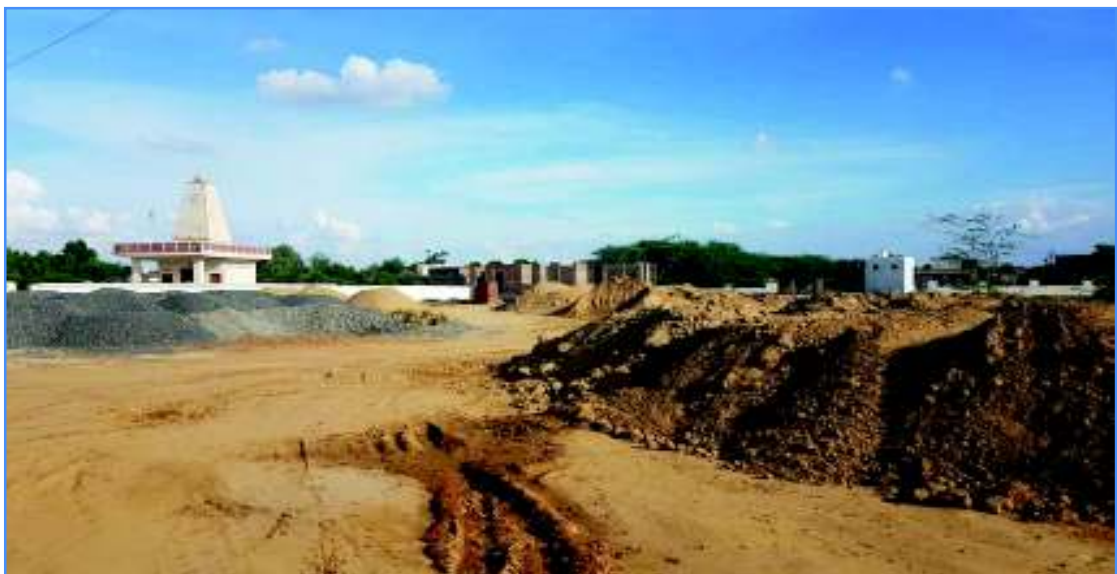
Photographs showing that no HT Line is passing from the proposed site.
