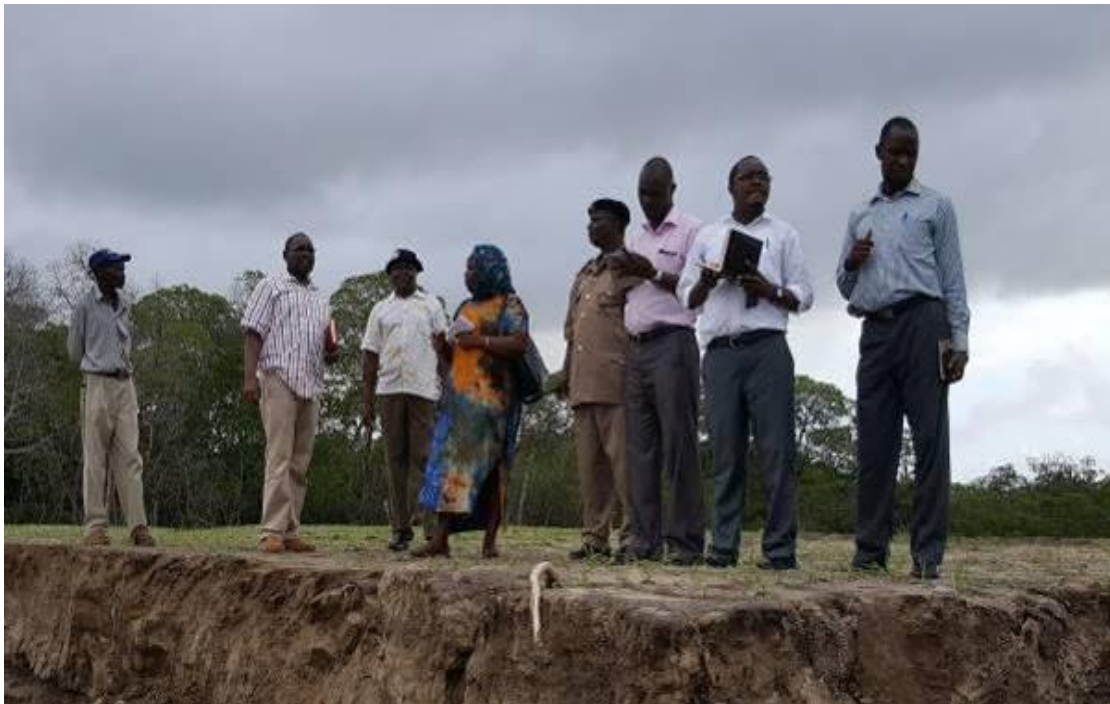
Plate 12: Consultants Undertaking a Field Case Study on 24th May 2016 at the Lamu Port Construction Site under LAPSSET Programme
