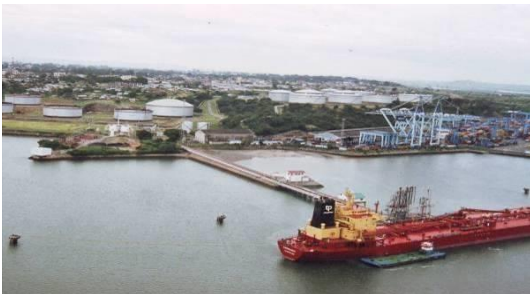
Plate 4: Product Receipt at Entry Point KOSF (Kipevu Oil Storage Facility) Mombasa Port
