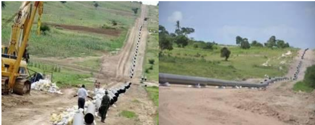
Plate 6: On-Going Construction of Mombasa-Nairobi Refined Oil Pipeline
