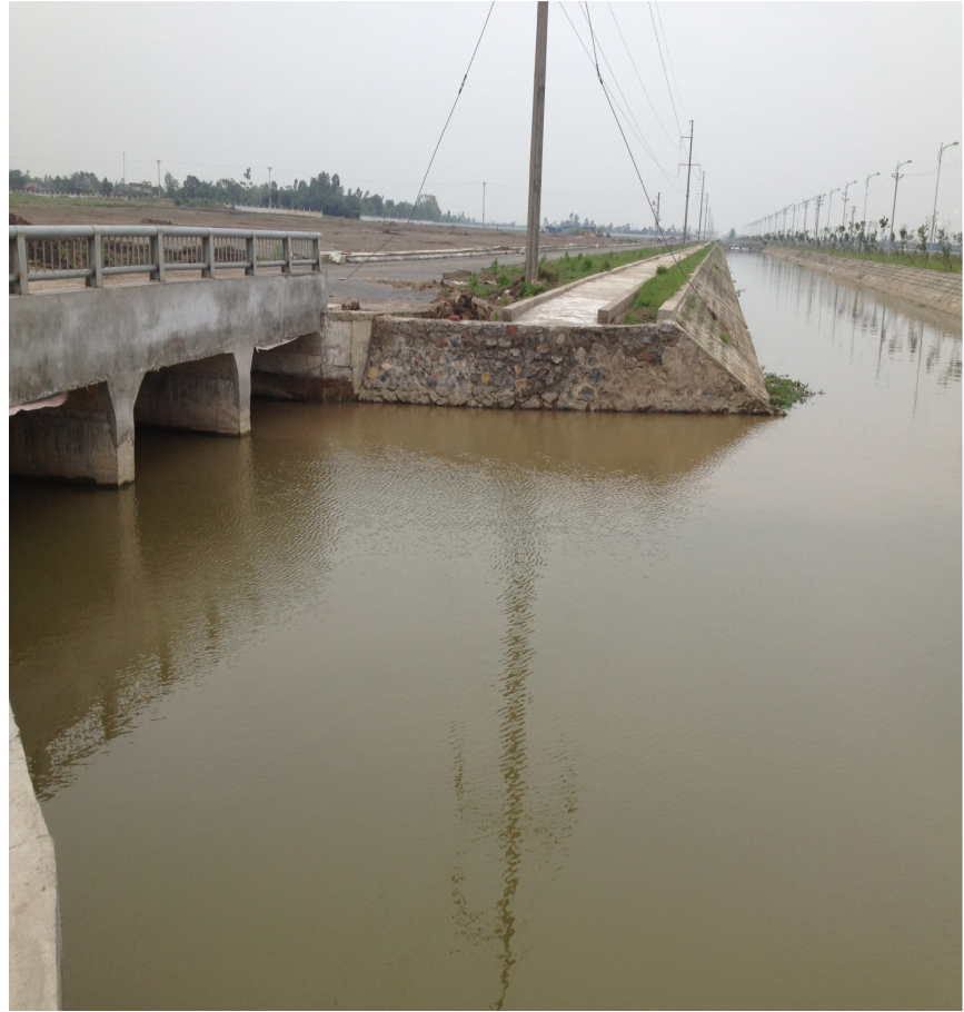
Sewerage network after processing in industrial zone
