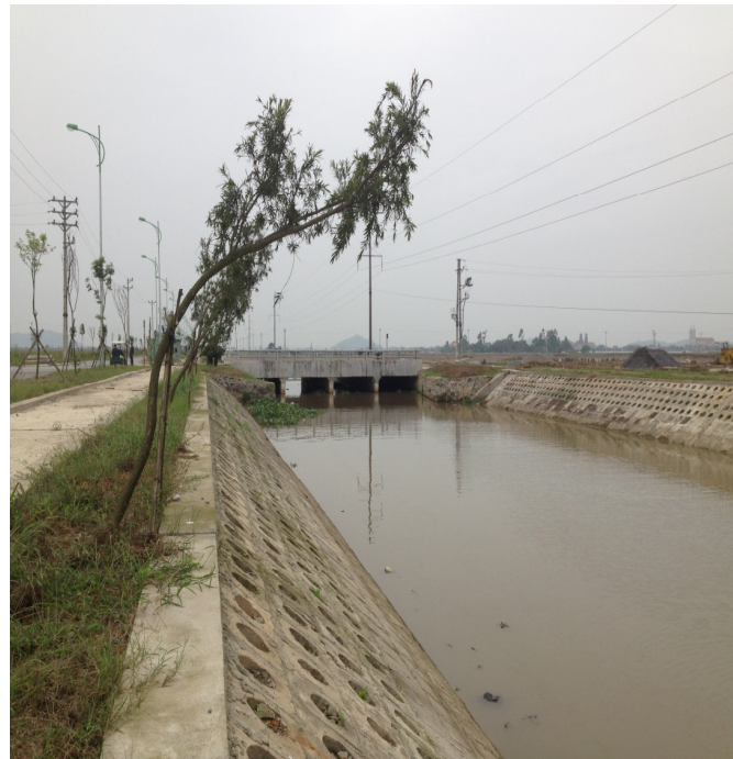
Location of effluent sewer in industrial zone
