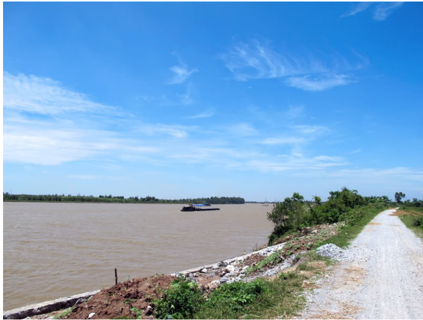
Figure 2-6. A part of Dao River crossing Bao Minh Industrial Park
