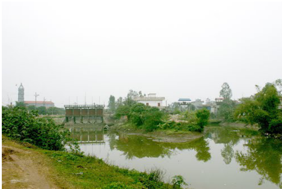
Figure 2-4. Sewer discharge to Dao River
