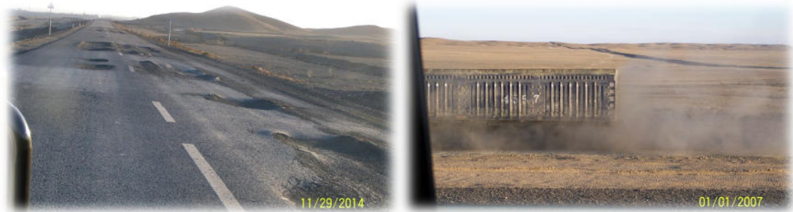
Figure 4.10: Coal transportation and road condition
