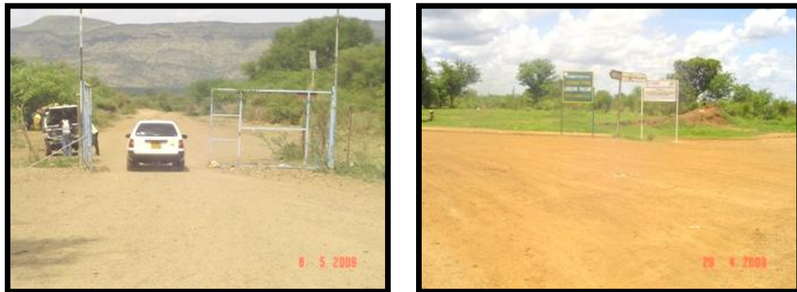
Plate 1: Beginning (0 + 000) and End Point (Nimule Junction)
