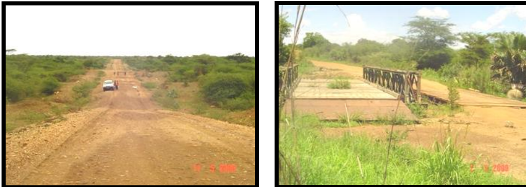
Plate 30: Sections of the Road and a Bridge
