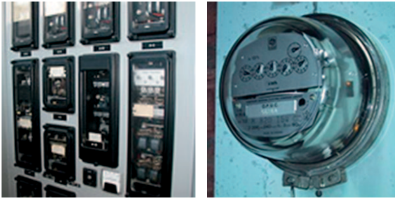
Figure 2.3 Electromechanical Protective Relays and Meters
