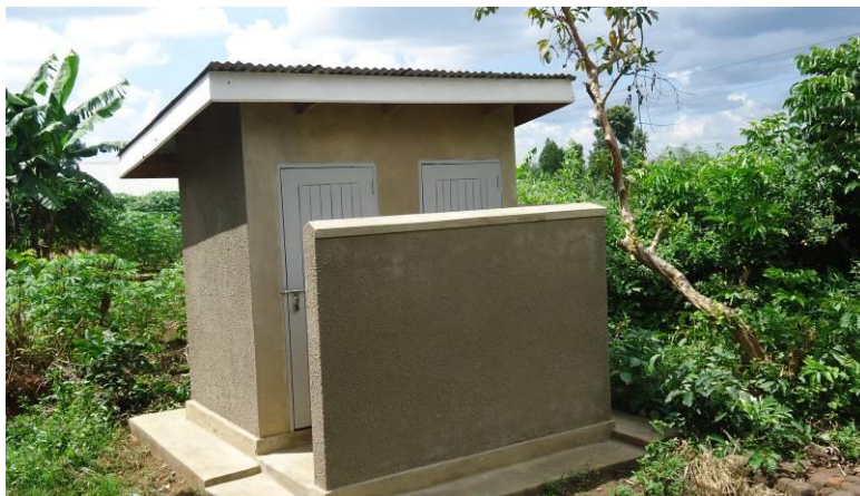
Figure 10-2 Latrine structure for a resettlement house
