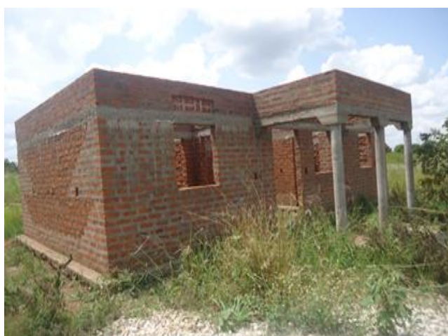
Figure 8-7 Residential house under construction in Namurwodho village, Nebbi
