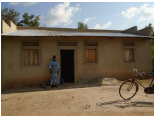
Figure 8-6 Residential house in Abilivillage, Gulu District
