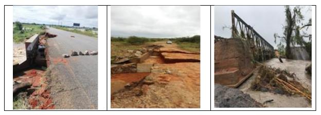
Figure 2: Impacts of cyclones Kenneth on road infrastructure in Cabo Delgado
