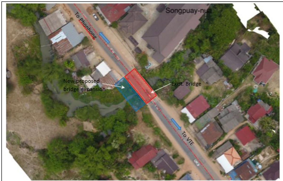
Figure 3-3: Nam Houm Bridge
