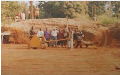
Nzerekore - Tile - Excavation
