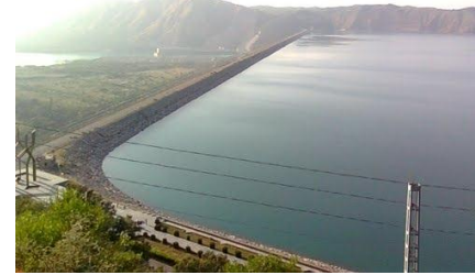
An Overview of Tarbela Dam
