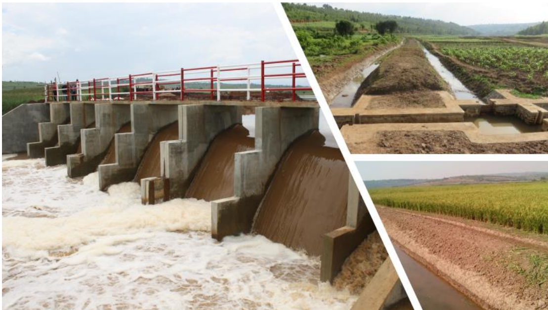
2: Typical water management infrastructures developed through the Project: dams, flow division structures, intake weirs
