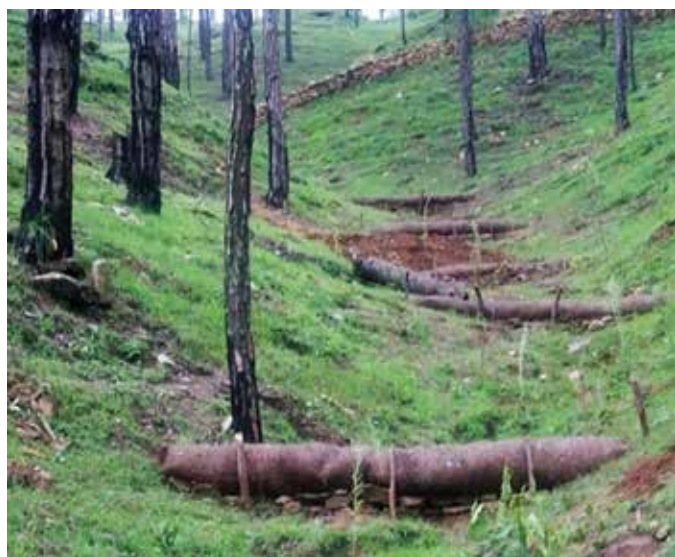
FIGURE 2.10: CHECK DAMS AND WATER RETENTION WORKS IN FIRE-AFFECTED CHIR PINE FORESTS OF UTTARAKHAND
