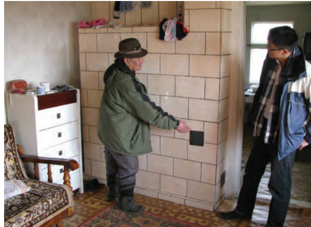
Back Side of Heating Wall
