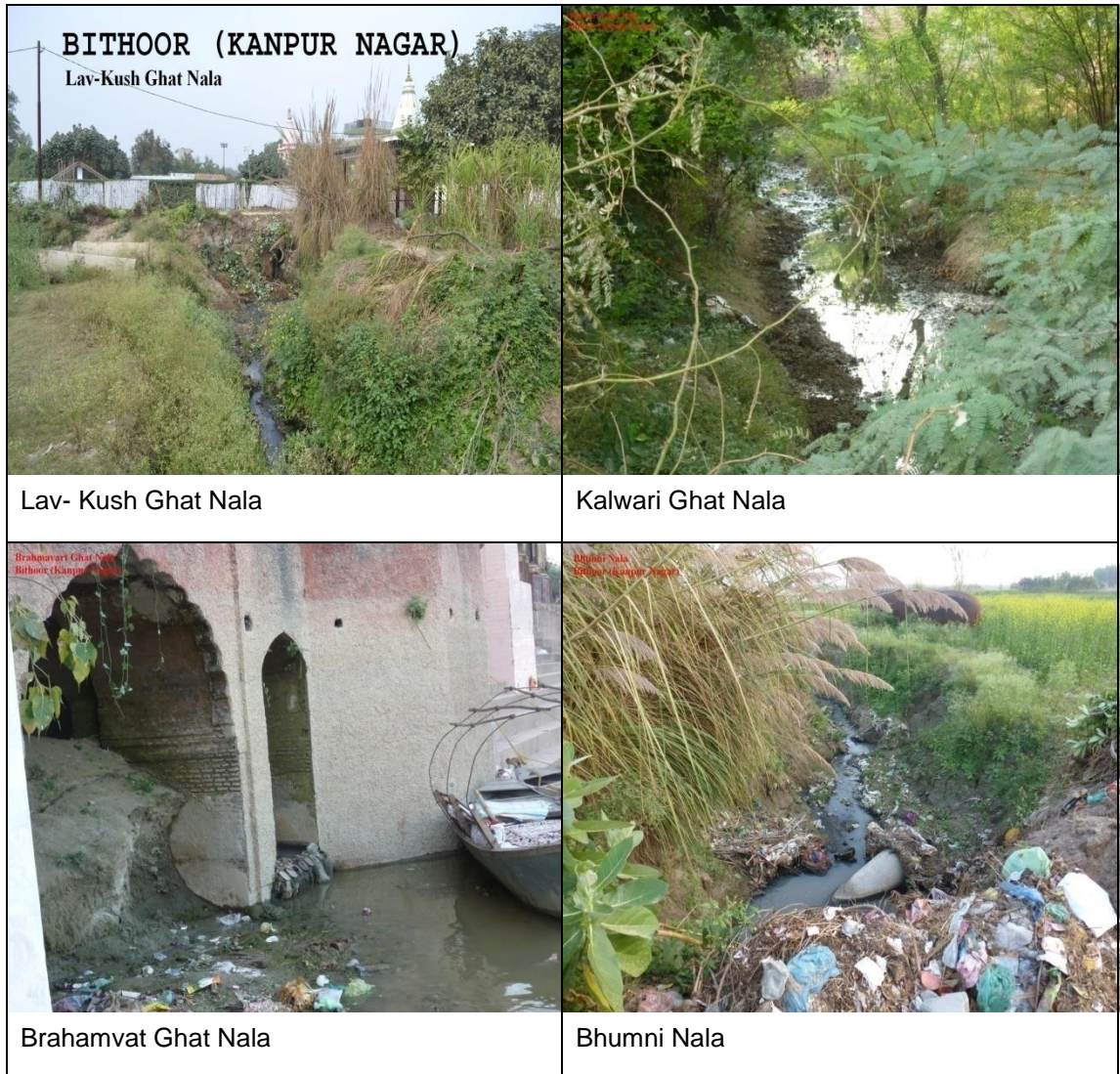
Figure 3-3 Photographs showing condition of Sewerage System of Bithoor Town
