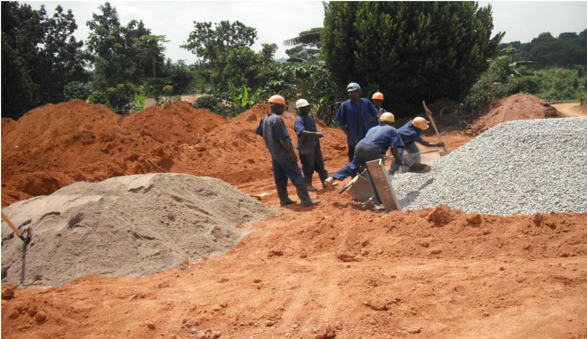
Plate 2.4: Construction of a lattice tower along Kawanda-Mutundwe line
