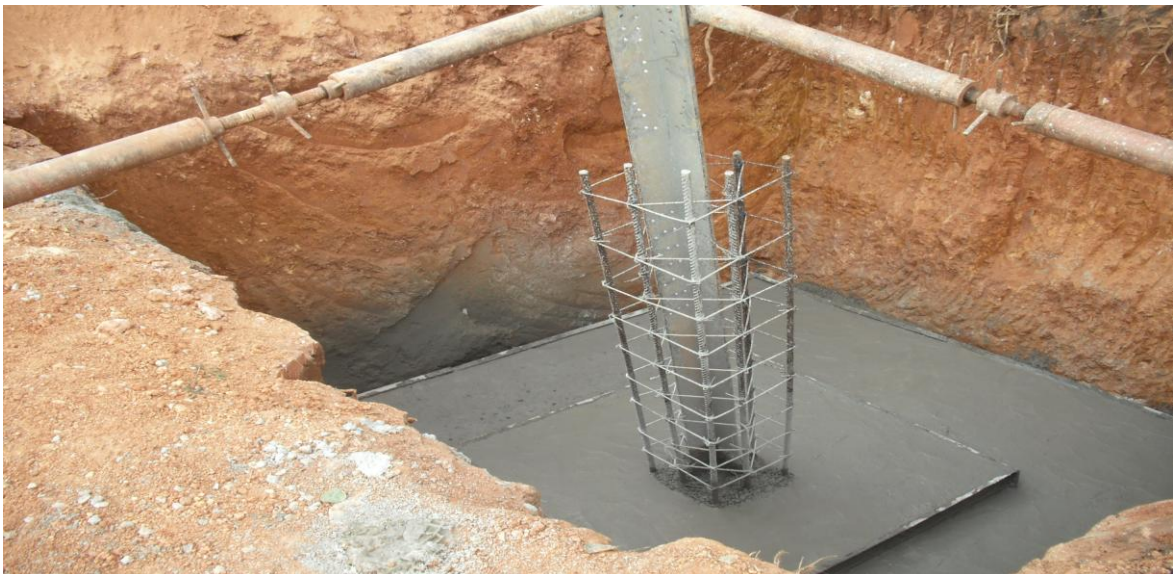
Plate 2.3: Pad and chimney Foundation for dry areas
