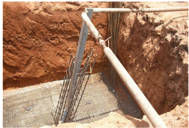
Plate 2.2: Pillar positioning and anchoring
