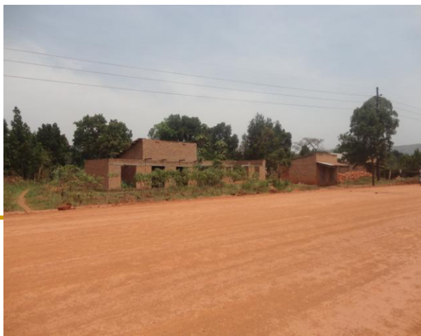
Transmission Line across Hoima & Masindi districts
