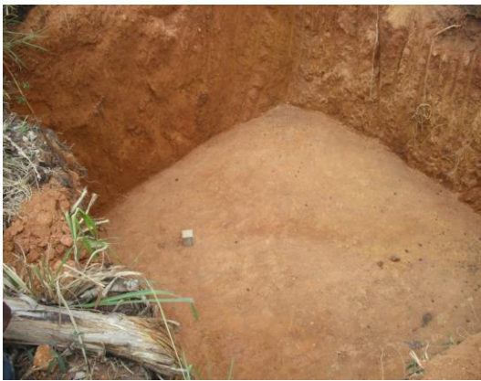
Plate 2.1: Foundation Excavation complete
