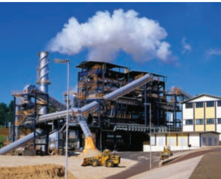
© Banco Itaú-BBA | The Santa Adélia in Jaboticabal in São Paulo, Brazil, a sugar cane cogeneration project financed by Banco Itaú-BBA (see story, p. 34). Residues of sugar cane production are used to generate clean energy for local energy distributors and the client's own use.
