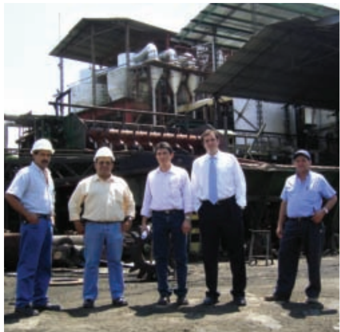
© Jouni Martti Eerikainen, IFC | The Ingenio la Magdalena sugar mill in Ciudad Merliot, El Salvador, financed by Banco Cuscatlán (see story, p. 38). The project design helped the company cut air pollution and waste water.
