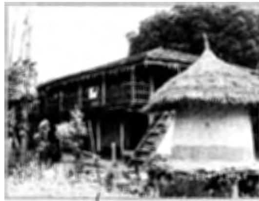
Affected House at Bengadabar VDC
