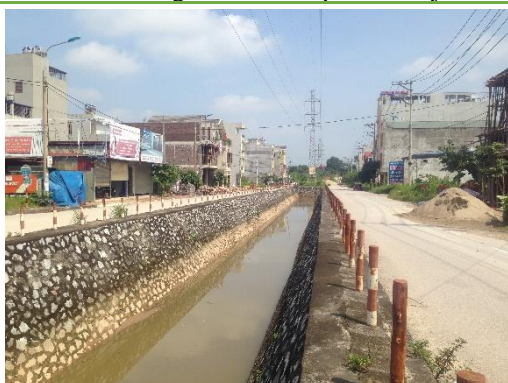
Change in ecological landscape after completion of ditch embankment (the embanked Mo Bach ditch section)
