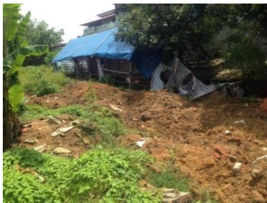
Xuong Rong drainage ditch area (Works No.6)
