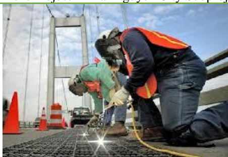
Figure 45: Reference image of welding activity when constructing the bridge
