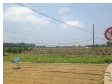
In the middle of Huong Thuong – Chua Hang road (works No.2)
