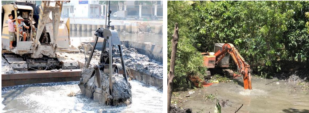
Figure 40: Reference image of sludge dredging from canals and ditches
