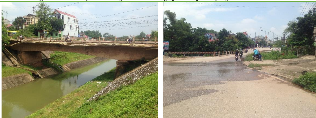
Figure 42: Traffic status at construction site of Dan bridge
