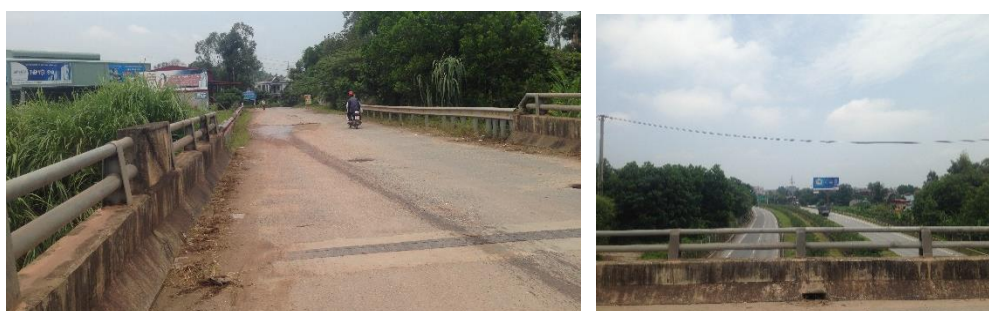
Figure 43: Traffic status at National Highway 3 overpass
