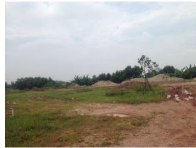
In the middle of Le Hu Trac road, nearby Highway 3 overpass (Works No.5)
