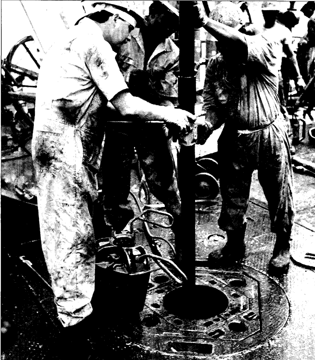
Running completion tubing on a drilling platform in the offshore oilfields of Benin. The countries of the region are demonstrating a heightened commitment to adjustment and policy reform.
