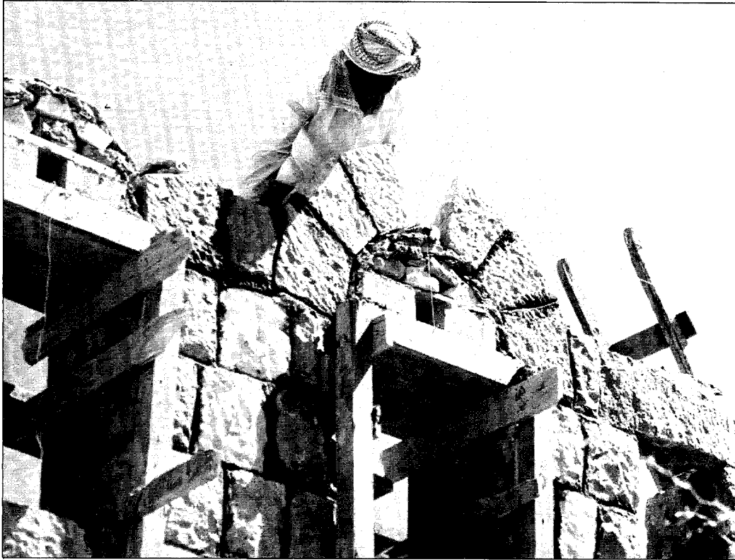
Stonemasons at work building a school near Sana'a, Yemen Arab Republic.
