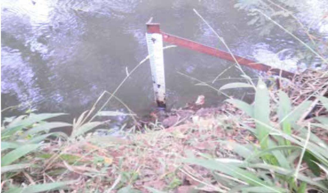
Figure 1.6 The 0 ó 1.5m Gauge Plate showing the rusted 0 - 0.6m section
