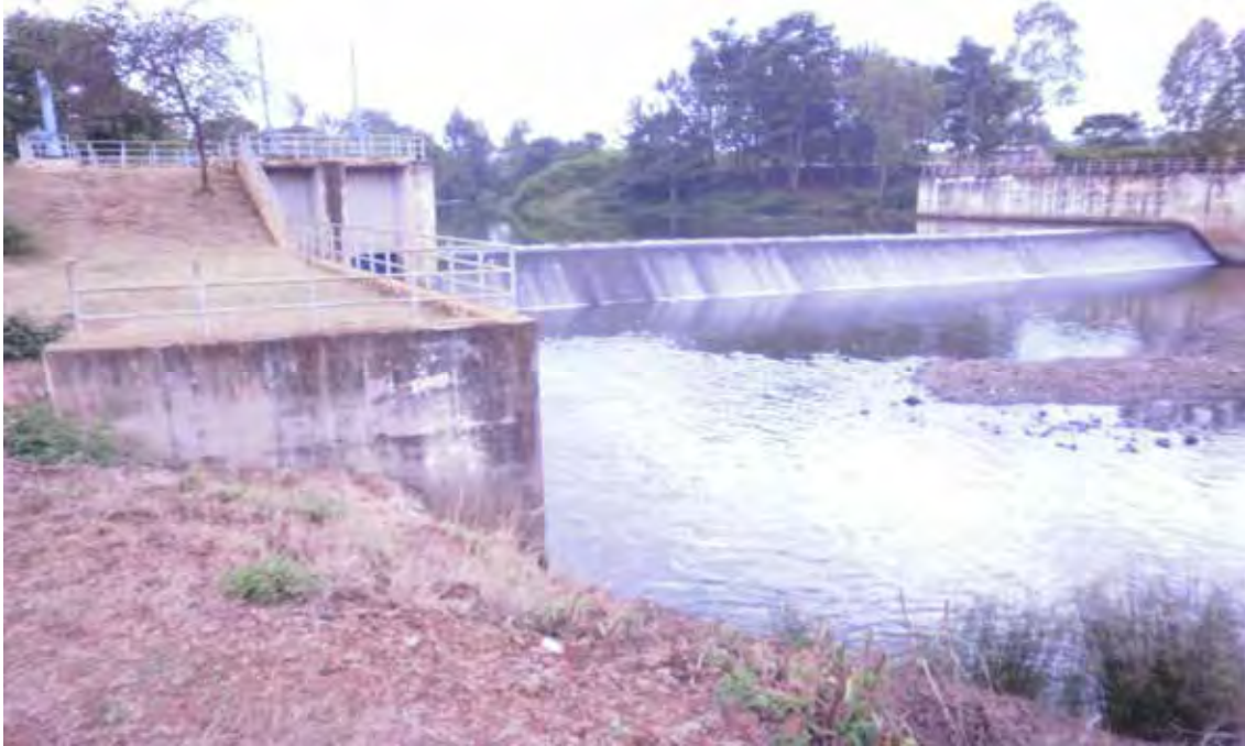
Figure 1.7 NIB Headworks Weir Transferring Nyamindi Flow to Thiba Basin
