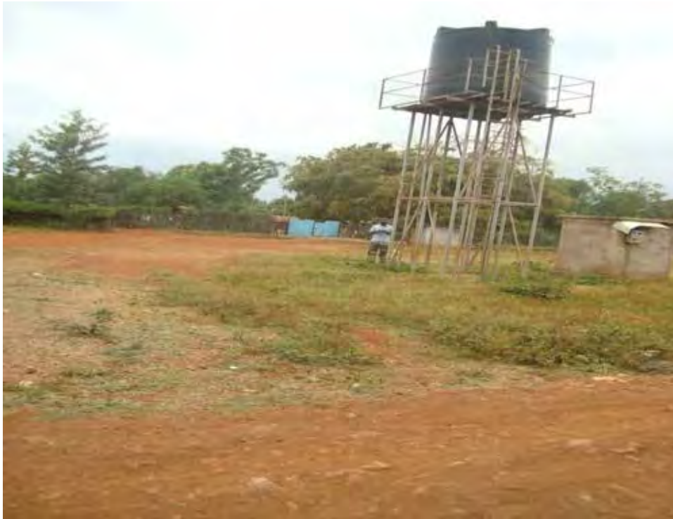
Figure 5 : Borehole at Gathigiriri village which was constructed through CDF but has never been used after completion
