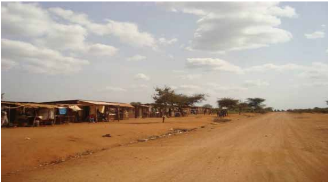
Figure 4 : Most of roads within the project area roads which are impassable during rainy seasons (Gategi - Makima Road)
