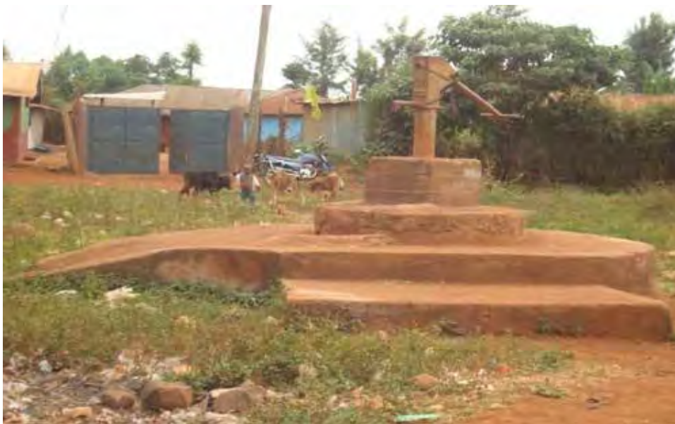
Figure 6 : Abandoned shallow well with a hand pump at Gathigiriri
