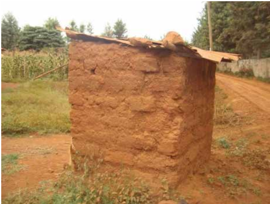
Figure 9 : Typical Pit Latrine in Gathigiriri village
