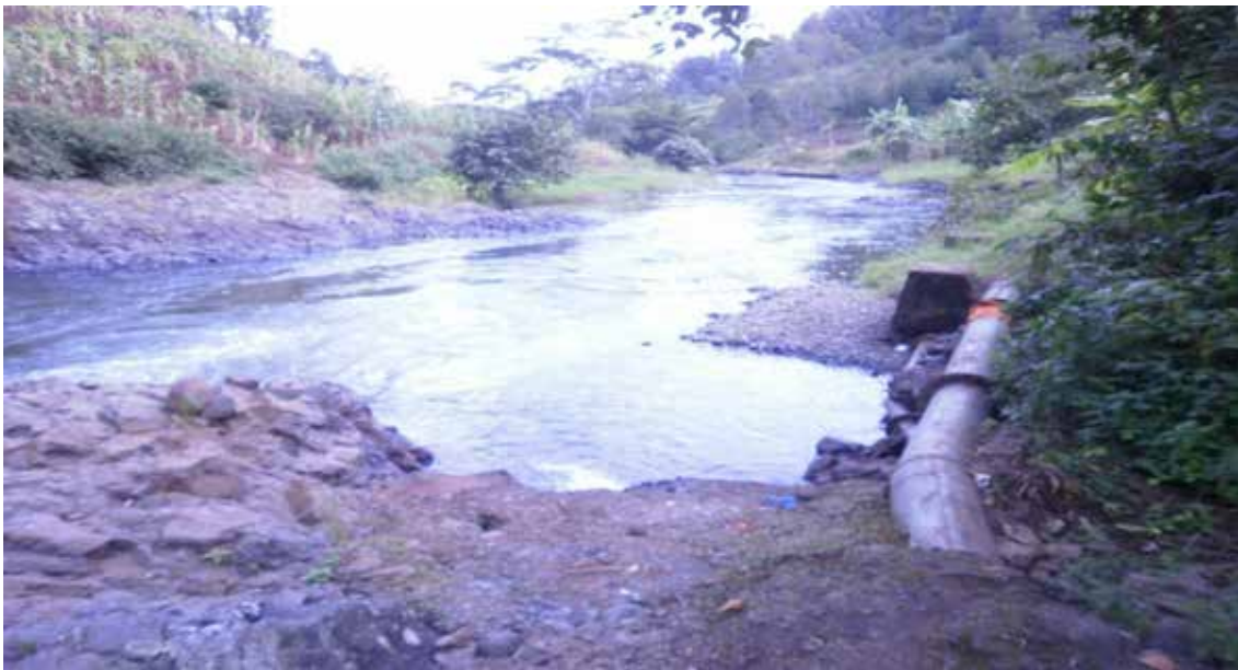
Figure 1.2 Kamumwe water intake site - about 100m downstream of Proposed Intake
