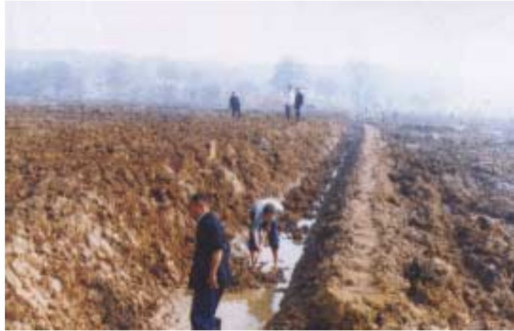
Branch Canal Repairing Under WUA Management
