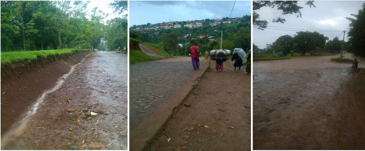
Plate 13: R2 serving the RDF Detach and Huye District Offices and R1 and R3 linking to National Road
