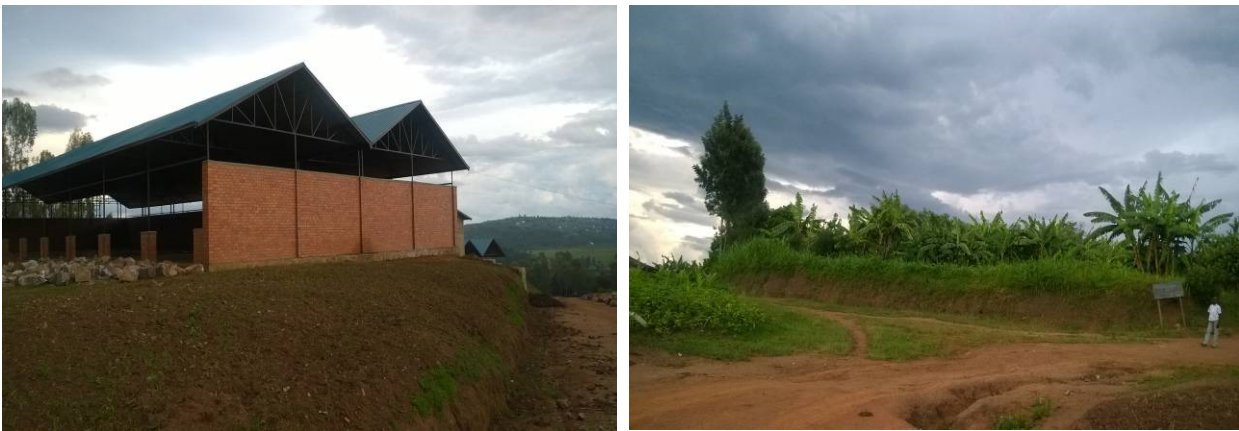
Plate 9: R19 and R85B will give access to the Handcraft Center, Mpanda Vocational Training Center and the proposed Muhanga industrial park
