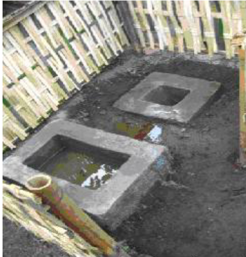
Concrete flush latrine with no air trap. Reservoir available for flushing and anal cleansing, Megaluh district, August 2007
