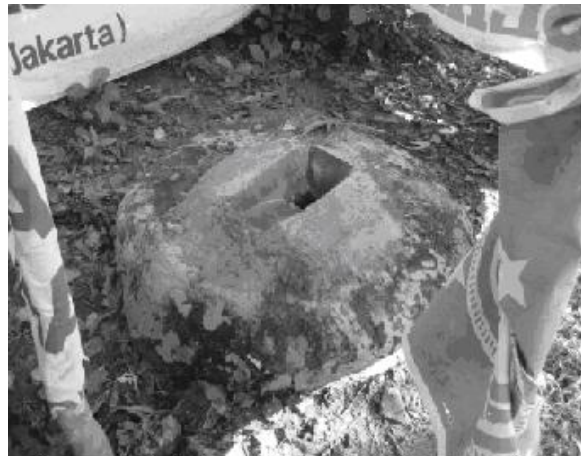
Unimproved pit latrine with plastic “walls” exposed to flies, Jombang district, August 2007
