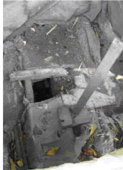
Simple pit with wooden plug and coarse log surface, Jombang district, August 2007
