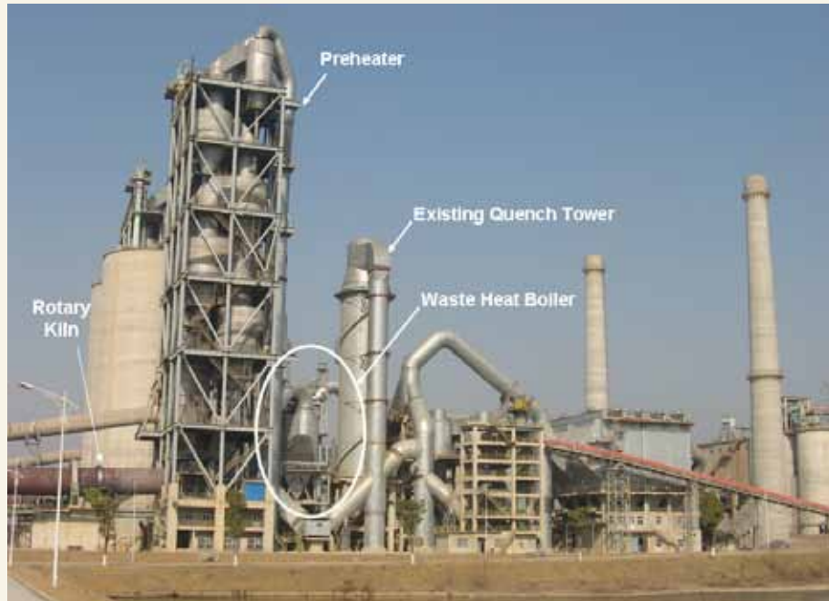
Figure 5: Preheater Waste Heat Boiler
