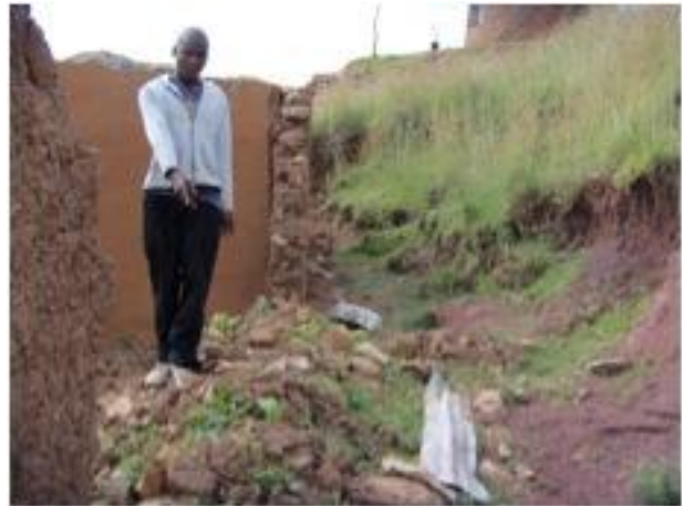
Figure: Weak anchoring of roof at some of the concrete houses in Kolonyama (Leribe); (right) Hill side run-off weakening and damaging mud / stone wall
