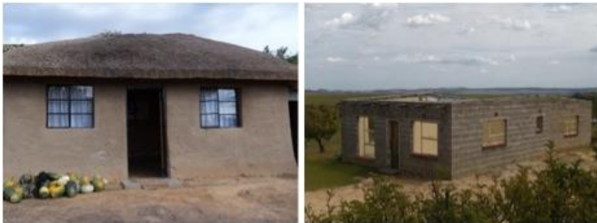
Figure: (left) Traditional heisi house type, built of mud bricks and Stones; (right) De-roofed bungalow type of house in Kolonyama (Leribe district)
