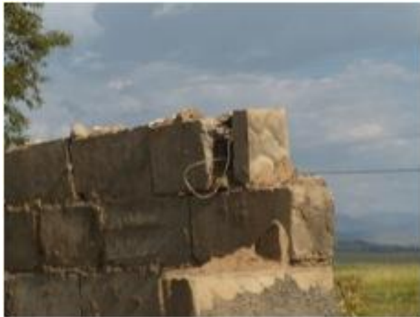
Figure: Weak anchoring of roof at some of the concrete houses in Kolonyama (Leribe); (right) Hill side run-off weakening and damaging mud / stone wall
