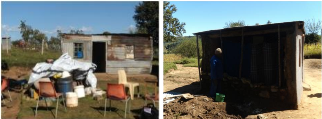
Figure: (left) Household storing remaining furniture from destroyed house under tarpaulin, background temporary housing made from corrugated iron in Ha 'Esekelo (Berea district); (right) Local reconstruction efforts, rebuilding mud / stone walls of polata (mud) houses in Serupang (Leribe district)
