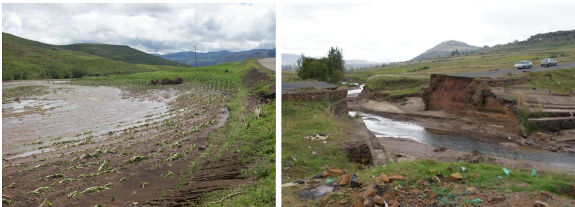
Figure 2: (left) Maize field water logged at Thaba-Tseka; Source: DMA Rapid Assessment Mission ; (right) Multiplate culvert washed away at Kubetu along B24 Road
