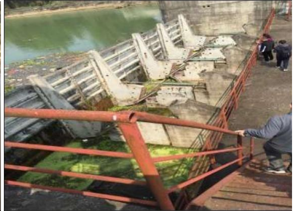
Gates at Xiadao Hydropower Station
