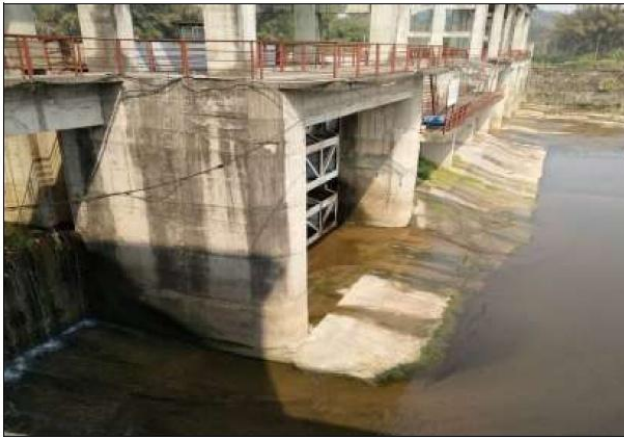
Dam at Xiadao Hydropower Station
