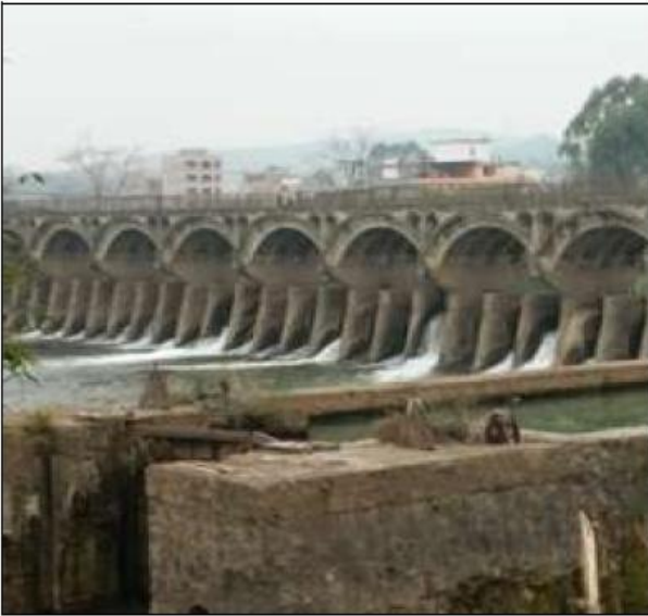
Dam at Fanglin Hydropower Station
