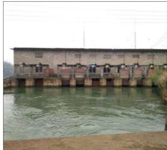
Water Gate at Huangshi Hydropower Station
