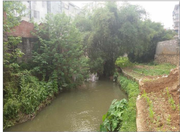
Huangansi Drainage Canal
