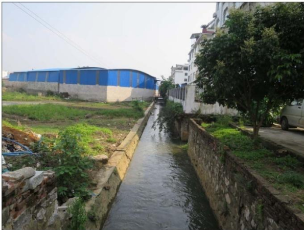
Shizigang Drainage Canal
