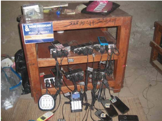
Solar charging station at Loma Mountains
