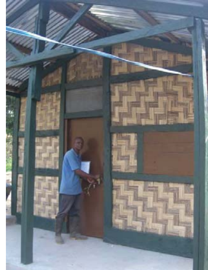
OKNP Site Manager with new eco-lodge
