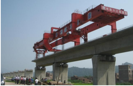
Picture 2. Beam Launching Equipment
