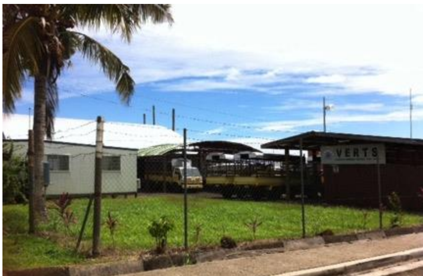
Figure 14 Existing block of land for NEOC office in Samoa
