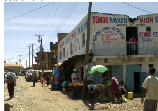
Figure 16: Electricity Poles on One Part of the Main Road, Which is Targeted for Improvement in Kayole Soweto Informal Settlement
