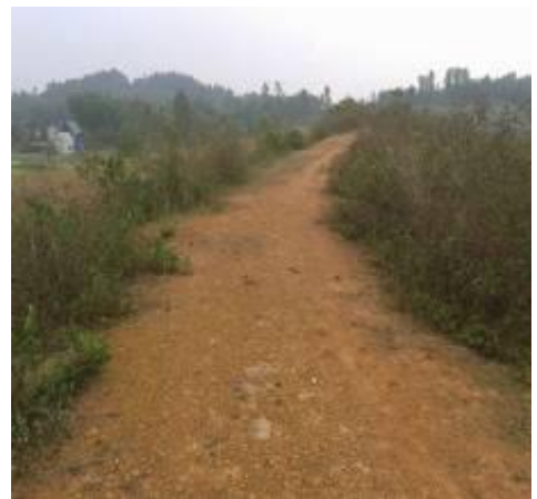
CURRENT CONDITION OF DAM CREST
