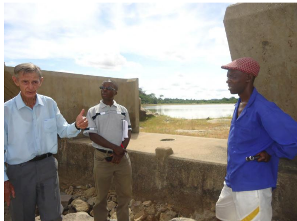
Ruti: Gap left by tipped fuse gate
