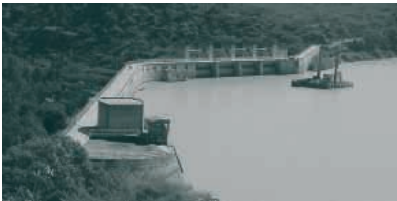
FIGURE 3.6 KOKA DAM – TACTICAL DREDGING NEAR DAM OUTLETS
