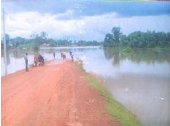
PR 2620 Flooded during Ketsana
