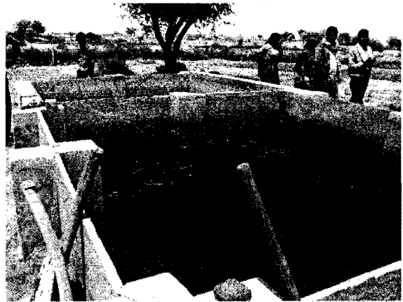
Water stored in Kund, Kunnu SHG, Jharira, Churu
