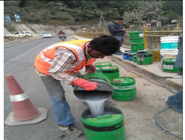
Repair (painting) works ongoing
