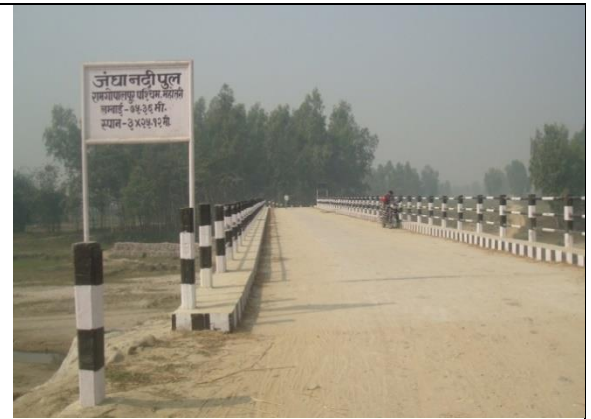
Completed bridge Jangaha river bridge
