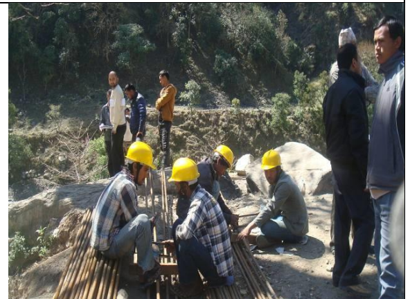
Workers on duty at Tipadagad bridge
