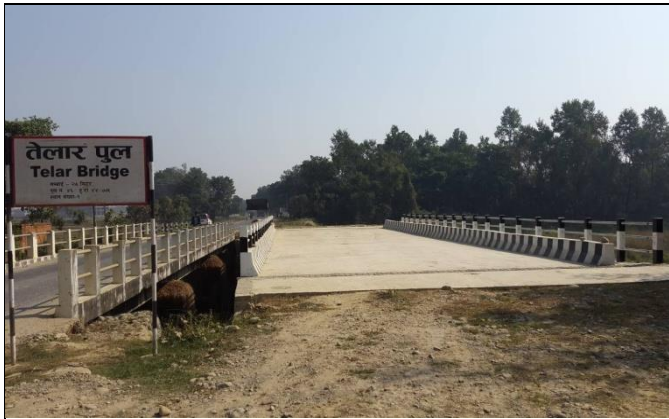
Completed Telar Bridge, Rupandehi
