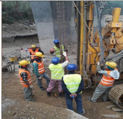
Workers on Major maintenance works at Jharai river bridge (45-H001-244)
