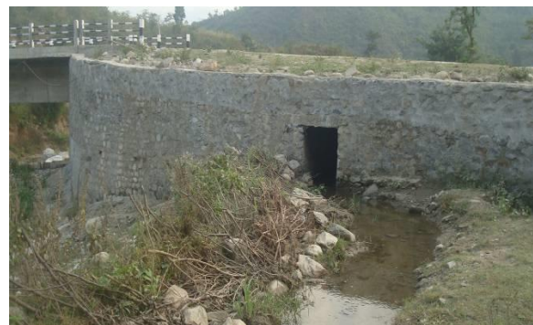
Reinstated irrigation canal, Kawa Khola Bridge
