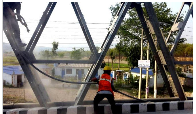
Sand Blasting work at Girwari Khola Bridge(45-H001-249)
