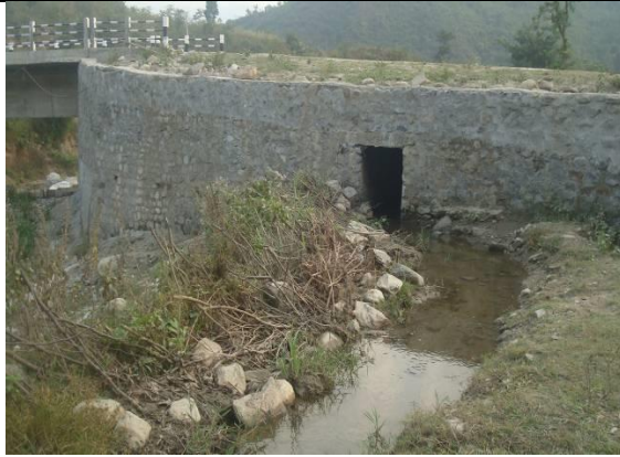
Reinstated irrigation canal, Kawa Khola Bridge
