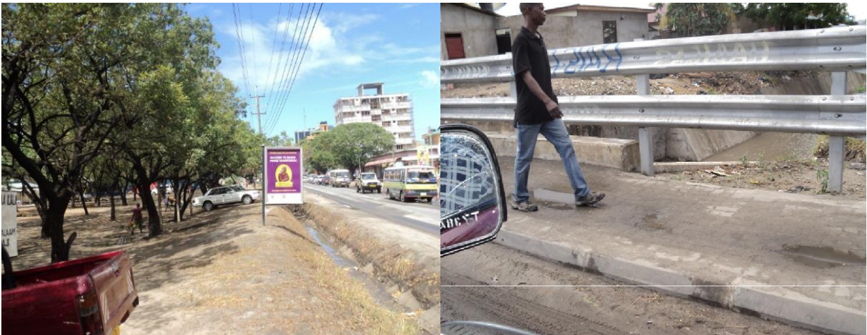
Figure 6: Project area showing some of the existing features including buildings, drainage system and light vegetation, along Uhuru road.
