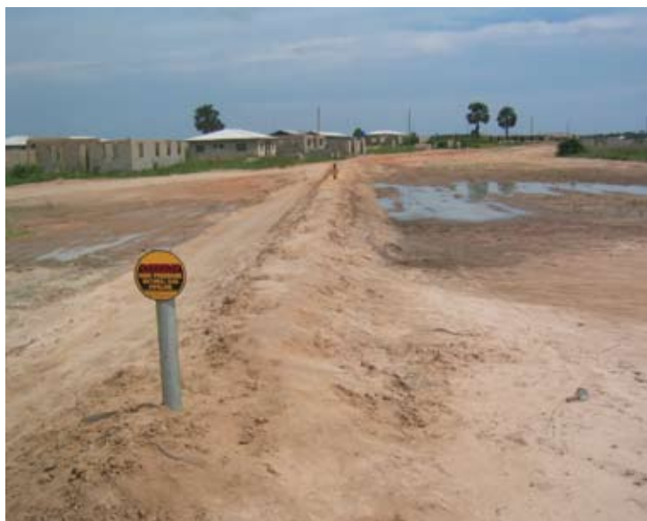
Nigeria: West Africa Gas Pipeline— Igbesa area
