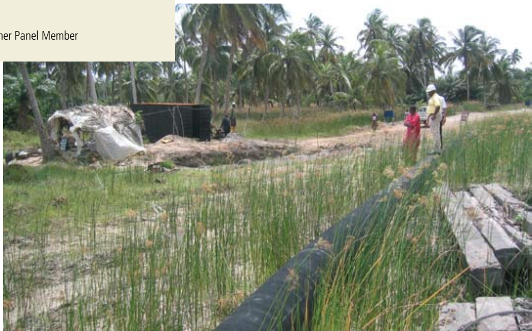
Nigeria: West Africa Gas Pipeline Project—Badagry area
