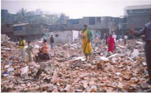
India: MUTP— Demolitions in Mumbai
