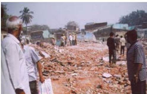
India: MUTP— Demolitions in Mumbai, India
