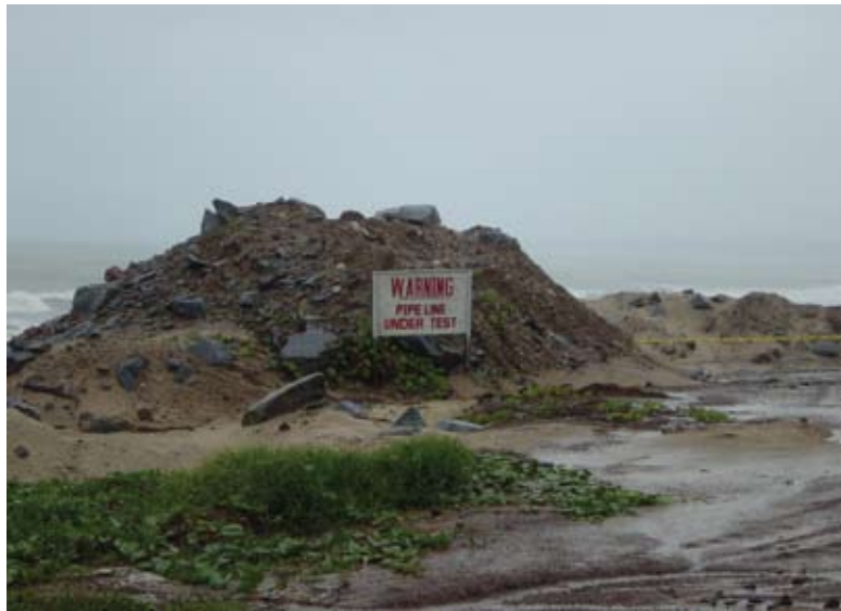
Ghana: West Africa Gas Pipeline— Takoradi area
