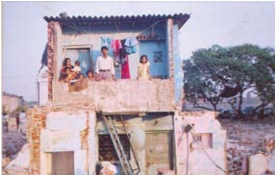
India: MUTP—House half-demolished as a result of road widening
