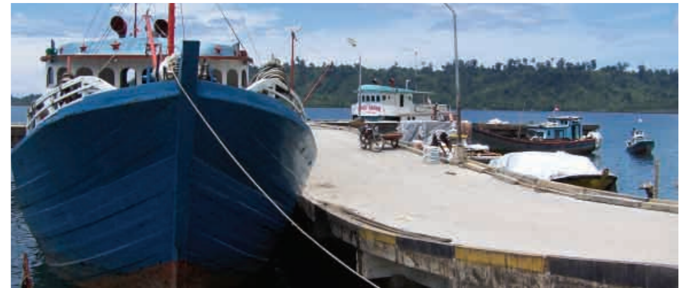
Rehabilitating the existing port in Sinabang
