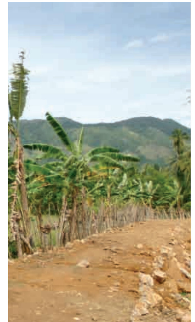
Reinforced village road
