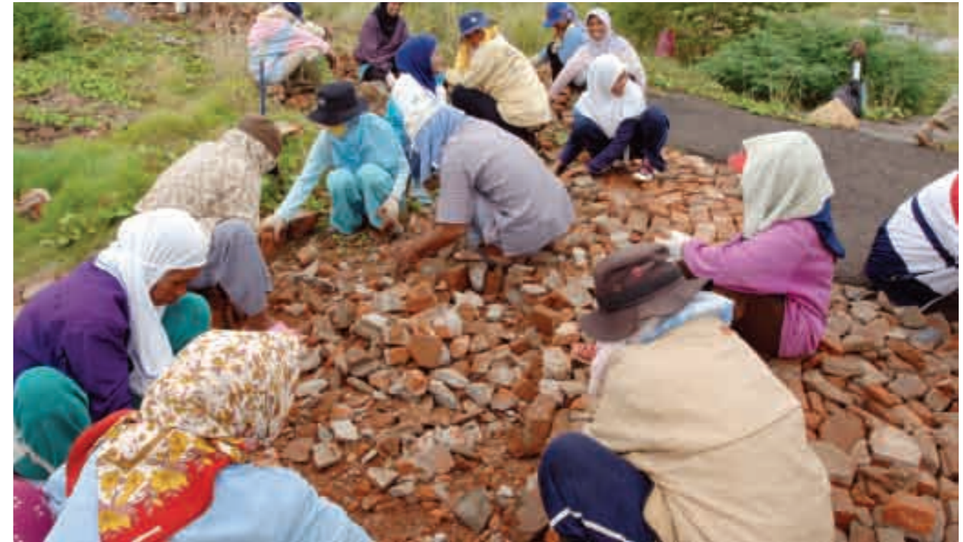
Tsunami rubble used to rebuild a destroyed road
