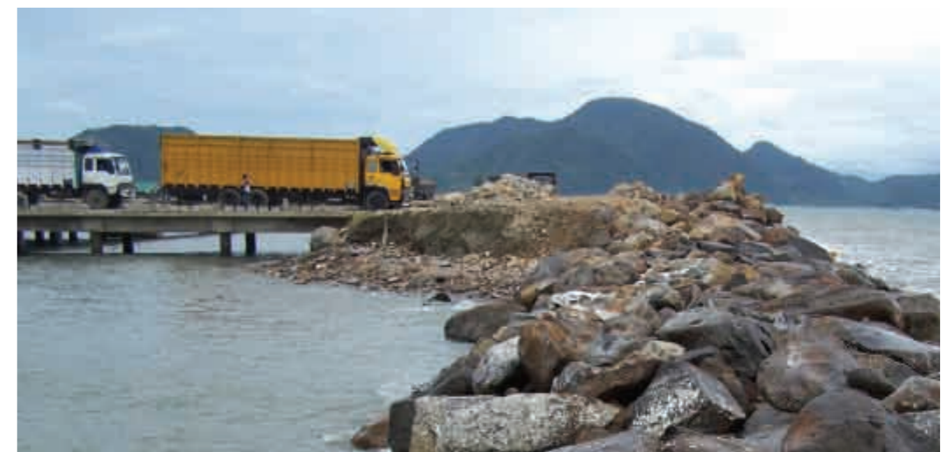
Port building site
