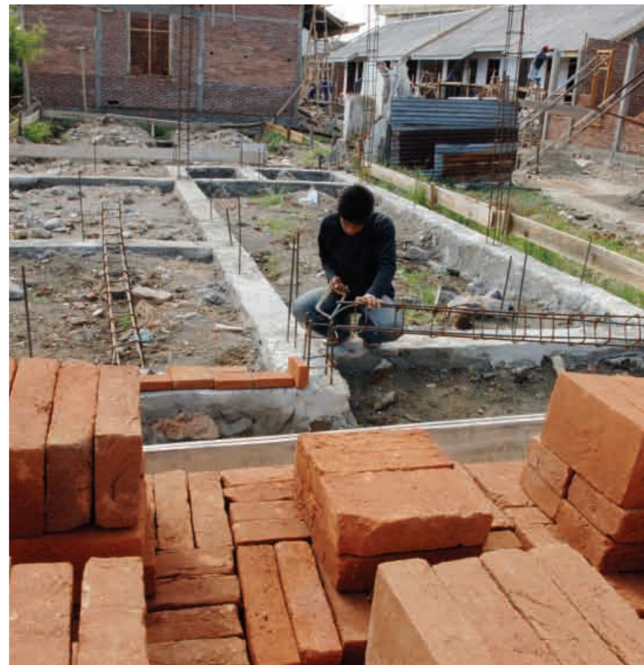
■ Ongoing construction in the Housing Project
