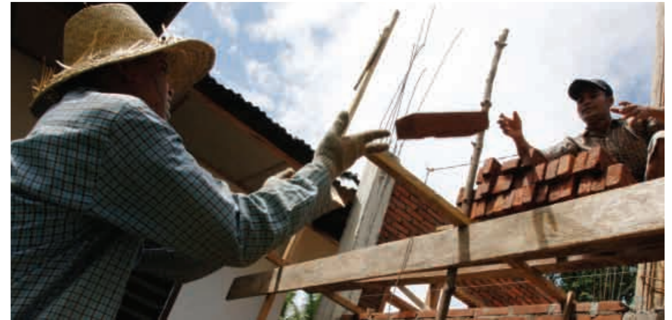
Workers in action - KDP community building their learning center
