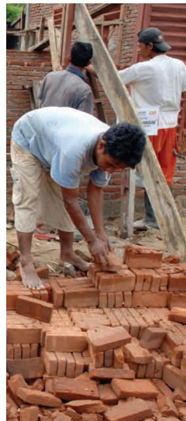
Enormous activity at the housing building site
