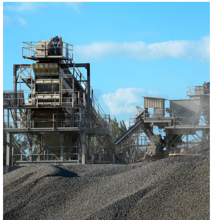
Basalt Rock Crushing in Mauritius
