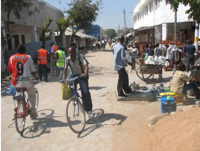
Plate 1: Existing road condition at the 6 th road sub-project.
