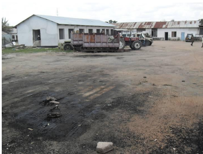
Plate 5: Existing conditions at the Municipal Workshop. Oil spills can be seen in the background
