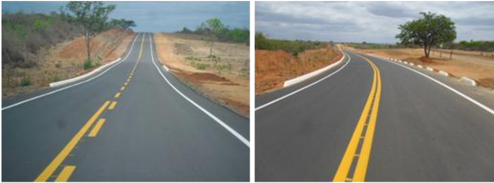
Pavement of the Road between Crato and Bela Vista
