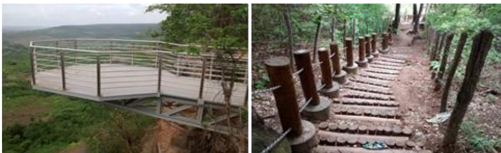
Infrastructure improvements in Geosite of Pontal de Santa Cruz
