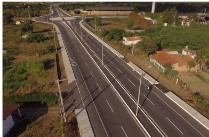
Section 1 of the Bypass in Juazeiro do Norte
