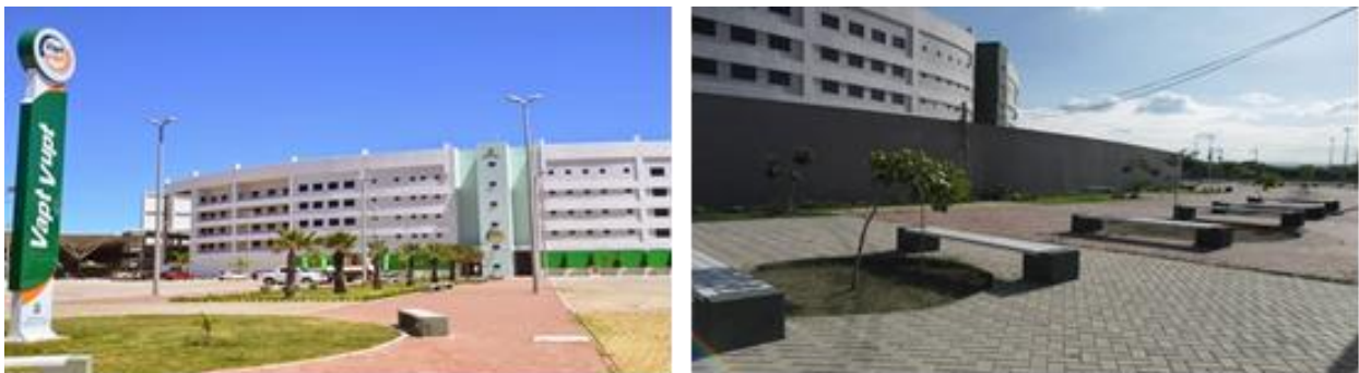
Multifunctional Center in Cariri
