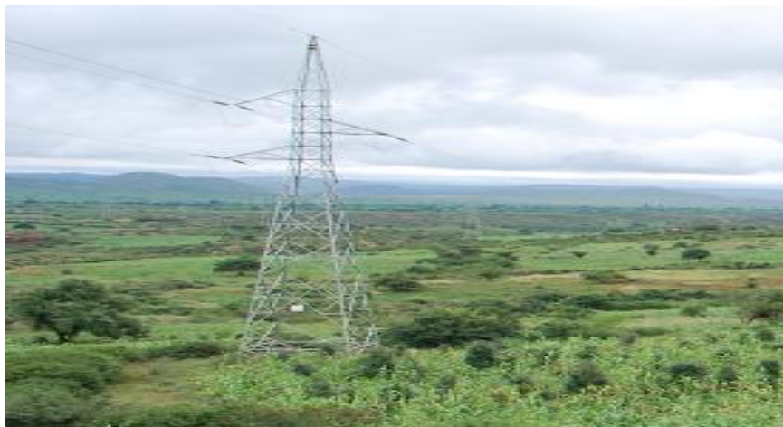
Figure 4. Facilities on site (electric power pole)
