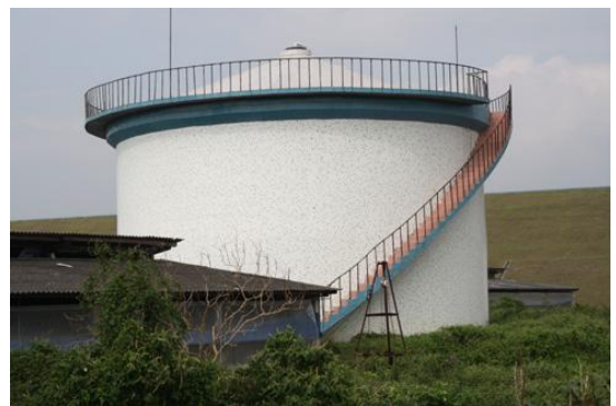
r. Biogas digester of Qishan Pig Farm, Chonglou Town, Taishan City
