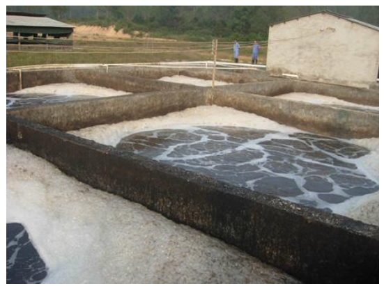
j. Aerobic treatment pool in Zhuangshi Pig Farm, Huicheng District
