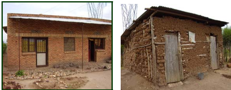
Photo of houses in the project area showing brick walled house and mud walled house.
