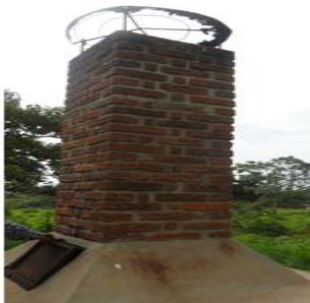
Picture set 2 – Sub-optimal health care waste management practice at a health care facility visited. Note that the incinerator is only two years old and is already showing signs of deterioration due to the load of waste incinerated. There is no waste minimization and segregation practices at the facility.
