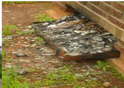
Picture set 2 – Sub-optimal health care waste management practice at a health care facility visited. Note that the incinerator is only two years old and is already showing signs of deterioration due to the load of waste incinerated. There is no waste minimization and segregation practices at the facility.
