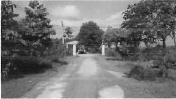
Picture 6. Entry to Tan Hung landfill and waste treatment site.
