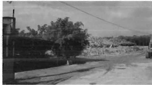
Picture 7. Tan Hung landfill and waste treatment plant
